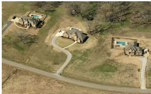
Large-lot single-family detached development is the primary character within Rural Residential areas (RR).
